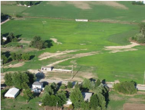
After the flood, Lola's house in background, the garage and foundation in the foreground.
