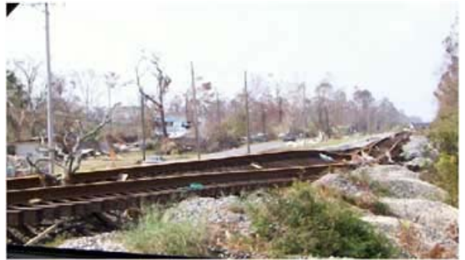
Not even the railroad tracks were spared
